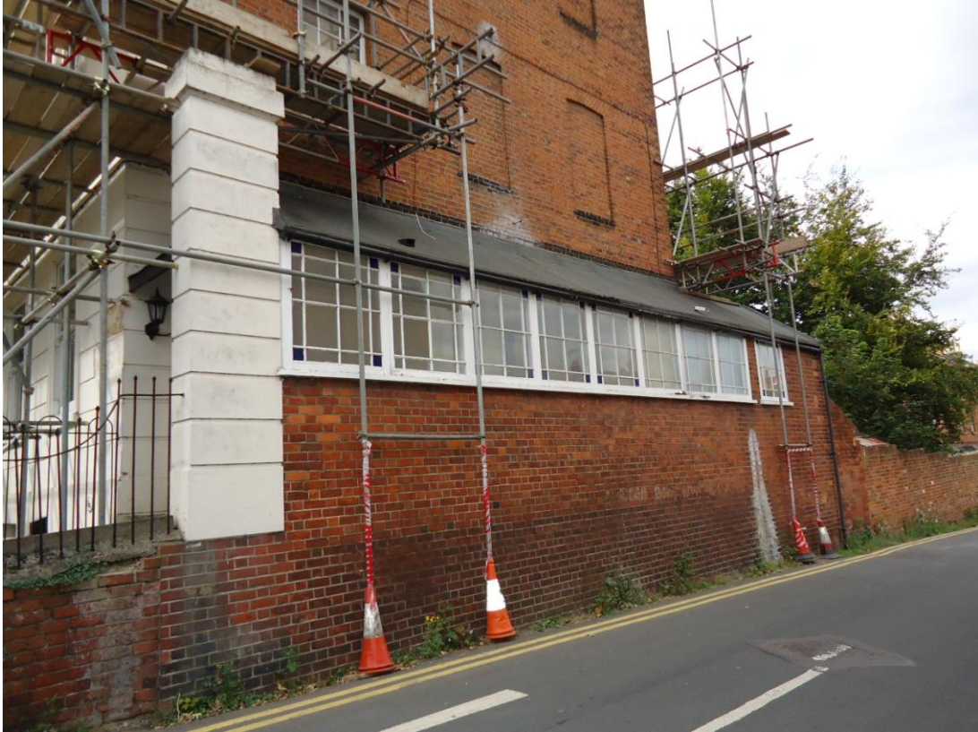
Walkway extension to East elevation (No access)
